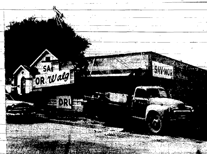
A BOOM TRUCK was required to hoist the sign in place for the new Sav-Mor Drug store at Tenth and Main streets. A segment of the sign is shown above being lifted into place. The drug store, now open, is owned by Dr. L. A. Jensen and Wayne Marsh. Workmen this week began blacktopping operations in the parking lot between the store and Arnie's Superette. The store will be managed by Roy Hinz, pharmacist, who moved here from Lincoln. His son, Charles, also a pharmacist, will assist him.
